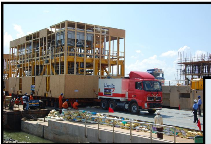
First heavylift shipment consist of 4 nos TEG Skid having dimension 19.20m x 8.48m x 9.0m – 159 MT rolled off from jetty in October,07
