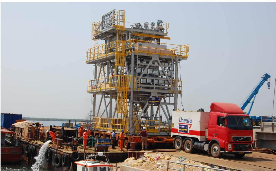
Package(PAU Centrifuges ) having height 13 m. loaded on barge Salina 1 being rolled off
