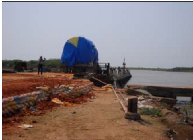
Jetty constructed at Machalipatnam
