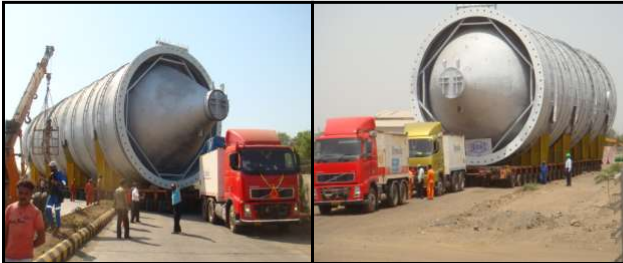
Transportation of Coke Drums having dimension 41.7m x 10.10m x 10.50m – 454 MT
